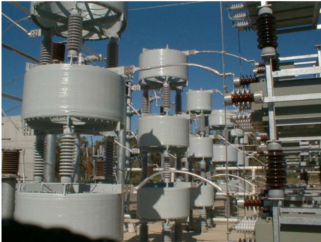
Fig.9.11 Typical industrial (HV) harmonic filters
